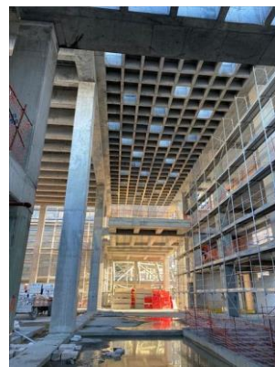
Figure 12. View from under the soffita (reinforced concrete cassette slab) towards the steel opera hall, construction phase (NTV, n.d.)
