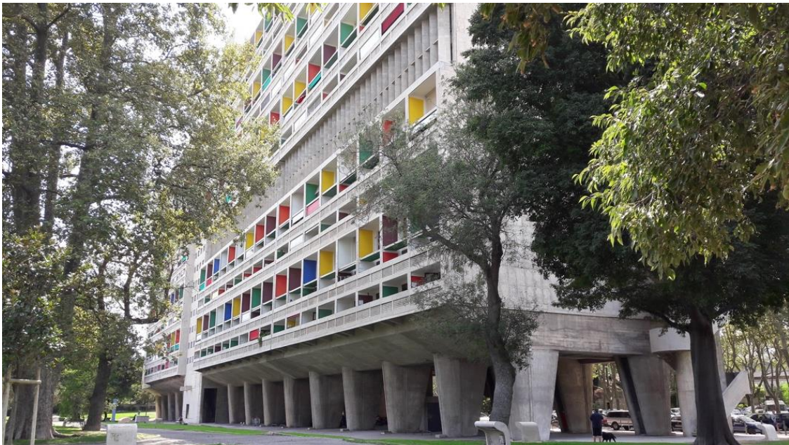
Figure 2. The Front Façade of Unité d’Habitation (Author, 2019)
