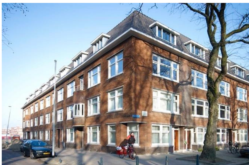
Figure 11. The Front Façade of Wallisblok (Hulshof Architecten, 2012)
