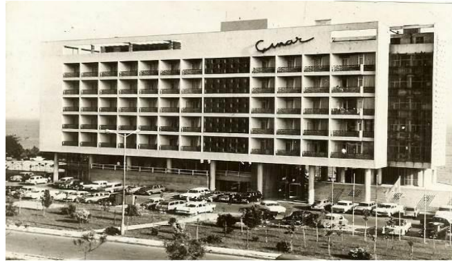
Figure 4. Çınar Hotel Entrance Facade -1958 (Böyük, 2008)
