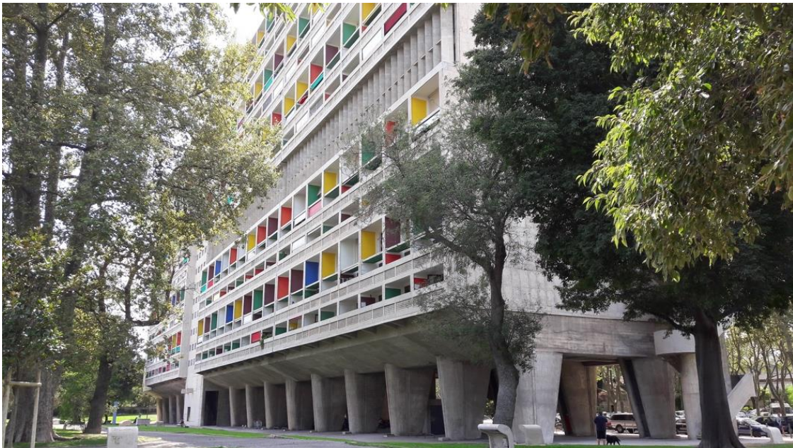
Figure 2. The Front Façade of Unité d’Habitation (Author, 2019)
