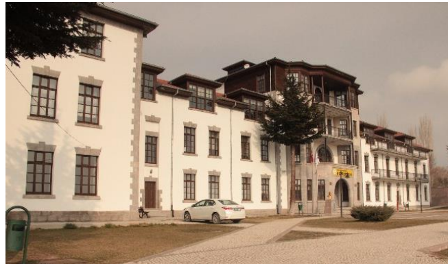
Figure 28. Anatolia College Hospital used as Merzifon High School for Science, taken from the east in 2019 (Gizem Özerol archive).
