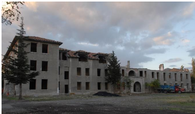
Figure 27. Anatolia College Hospital before the repair, taken from the east in 2005 (Sadi Bayram archive)
