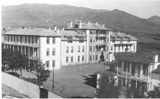
Figure 25. Anatolia College Hospital, 1900s, taken from the east. 28
