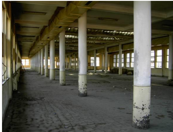
Figure 21. Production building (building 1) (competition statement, 2006).
