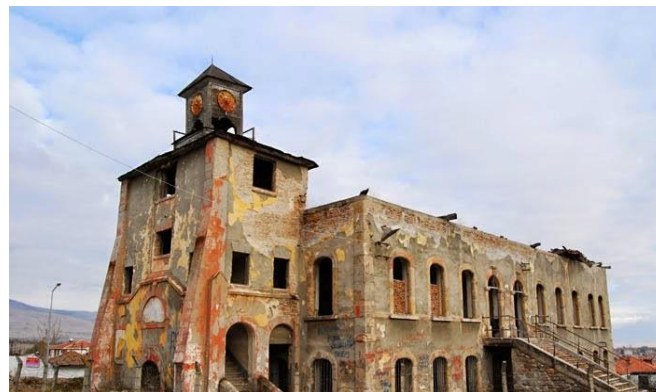
Figure 12. North College, taken from the south-west, before restoration. 19
