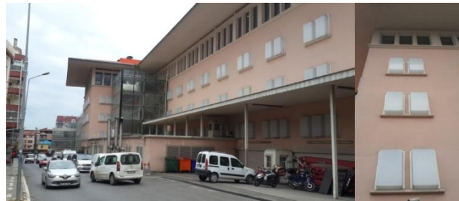
Figure 20. The Western facade and the window detail (Yusuf Bera Bilici archive, 2018)
