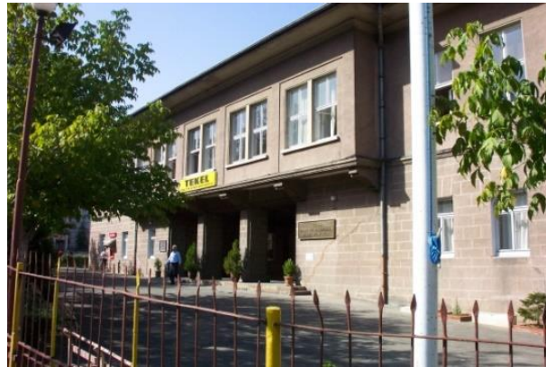
Figure 16. Building 1 before demolition, 2006 (Competition Statement, 2006)
