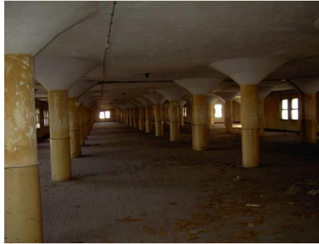
Figure 4. Building 3, flooring system (Competition Statement, 2006).
