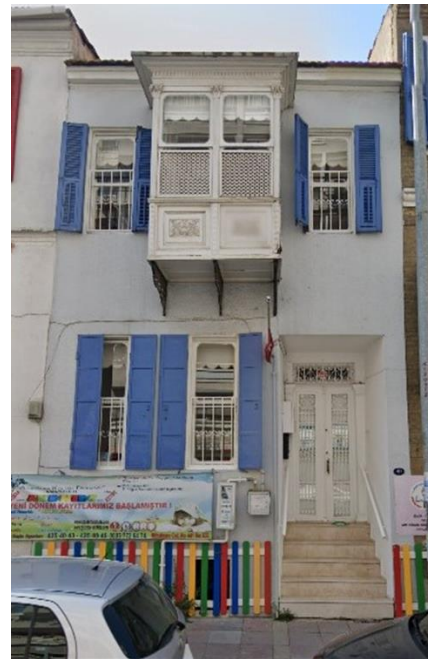
Figure 4. Classic Levantine House Facade from Konak (Author's archive, 2024)
