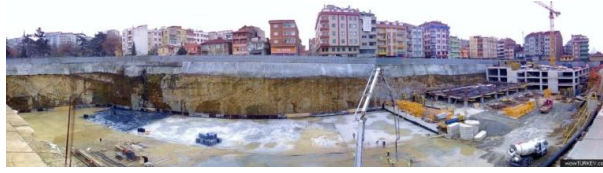
Figure 6. Trabzon Tekel Cigarette Factory land, construction phase 2009 (wowturkey.com photograph :Volkan Soner)
