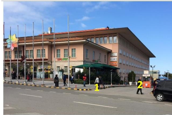
Figure 19. Shopping mall eastern facade (Müberra Kabataş archive, 2019)
